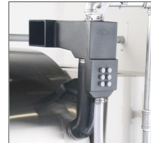
Safe chemical injection
